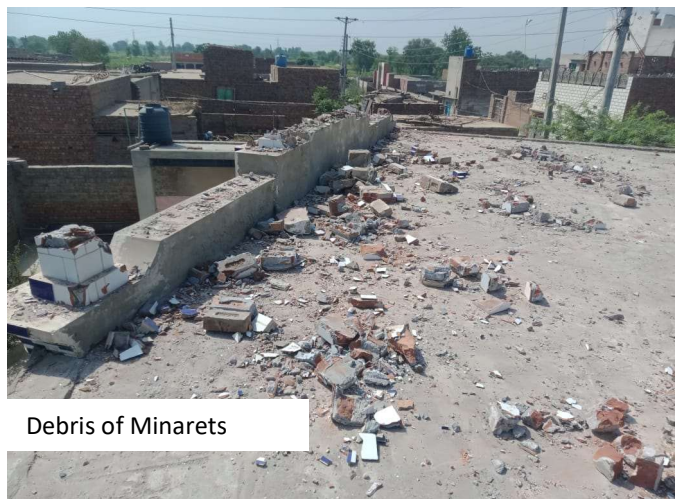
Debris of Minarets
