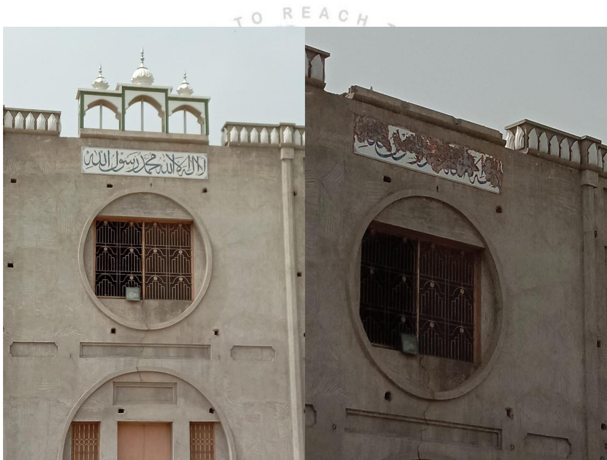
IMAGES BEFORE AND AFTER THE INCIDENT
